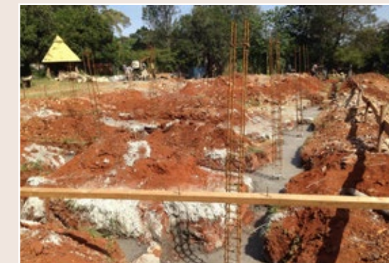
Baustelle in Langata
